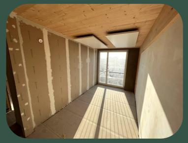
Ekopanely boards are 4 or 6 cm thick and typically mounted as sandwich wall on studs before plastering.
