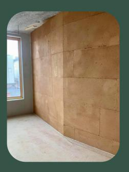
Lemix panels are 22 mm thick and typically mounted with screws before plastering with clay plaster.
